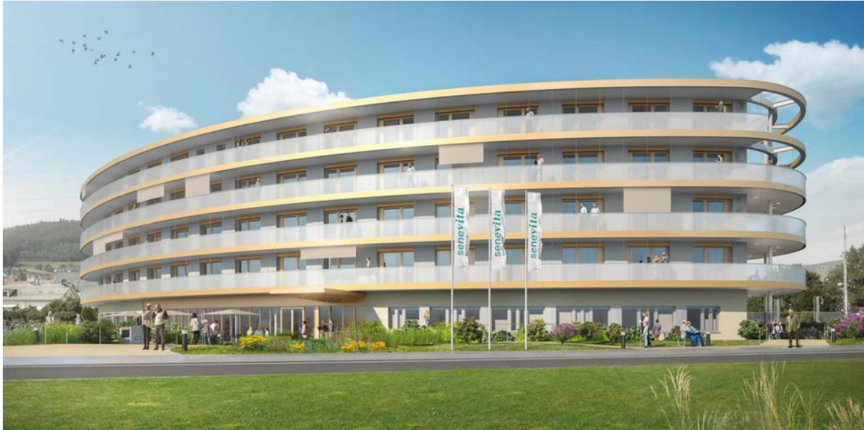
The Hycleen Automation System is suitable for new buildings such as the senior and care center Senevita Mülibach (Switzerland). Source renderings: Senevita AG
