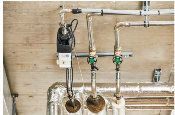
The Hycleen Automation System ensures optimum hygienic conditions in the long term due to the circulation system with automatic adjustment capabilities.
